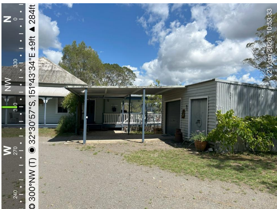
Photo 9: View of the carport adjacent to the eastern side of the residential dwelling.
