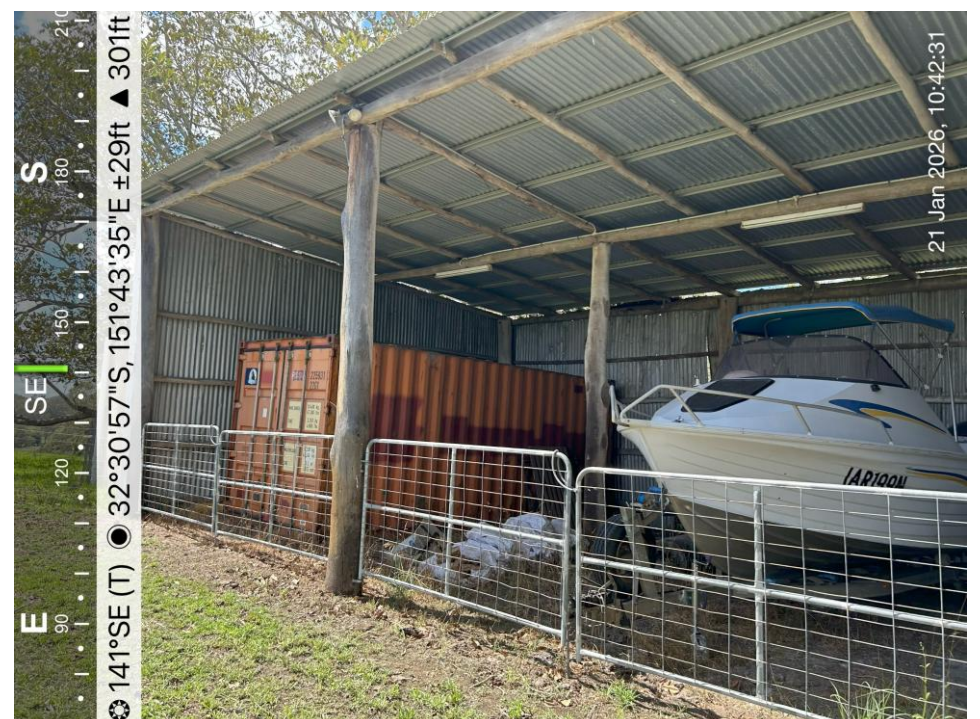
Photo 4: Overview of the shed located to the eastern section of the site, used for storage.
