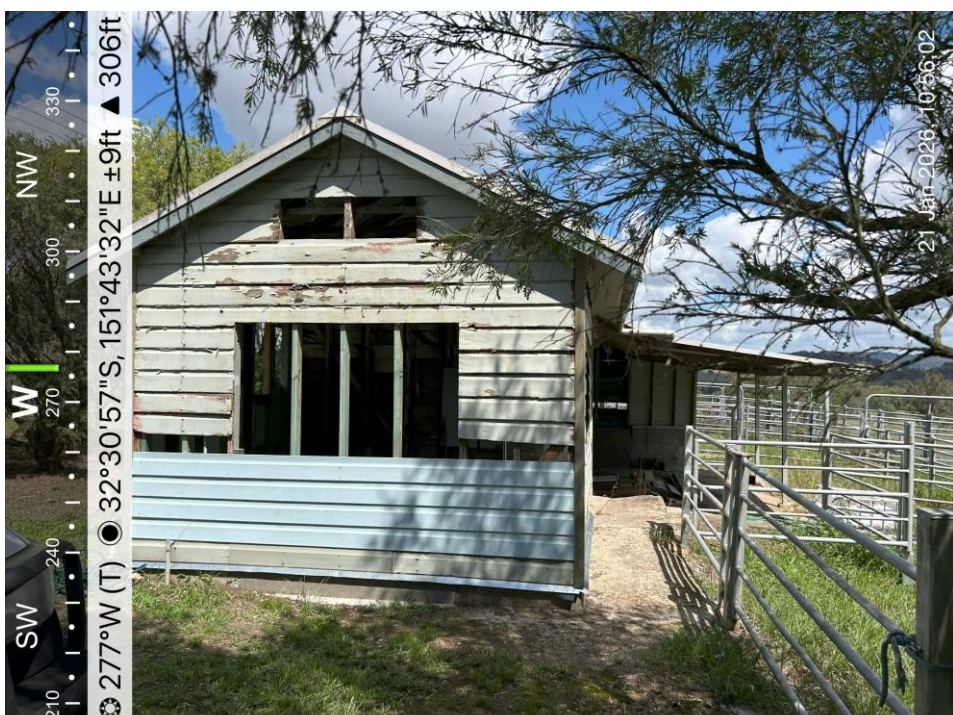
Photo 11: View of the livestock shelter located to the western section of the site.
