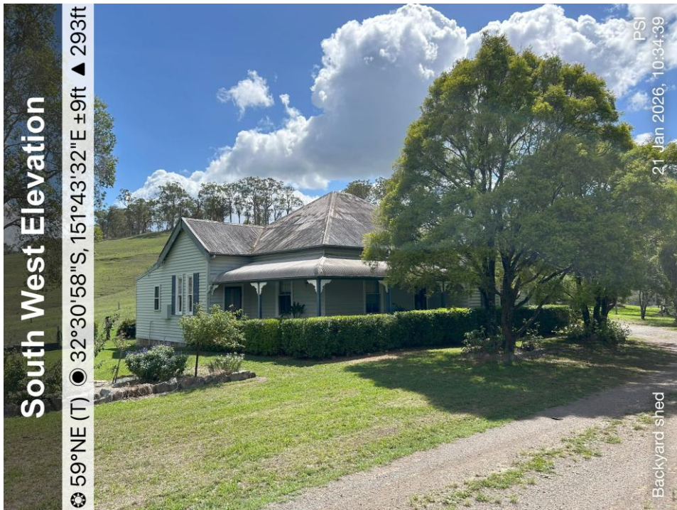
Photo 1: Overview of the residential dwelling.
